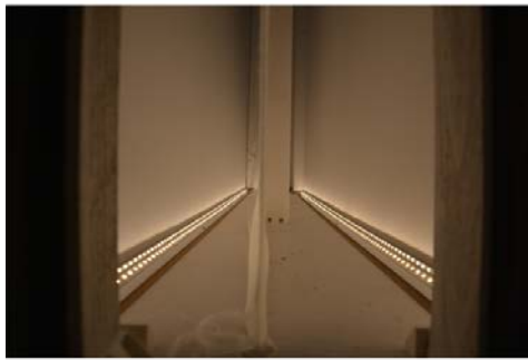
Installation of the VariWhite LED Tape at the top and bottom of each wall
